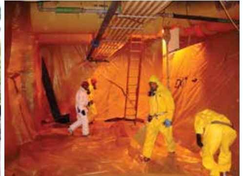
WPCS Step Feed Phase I, Akron, OH (Asbestos)
